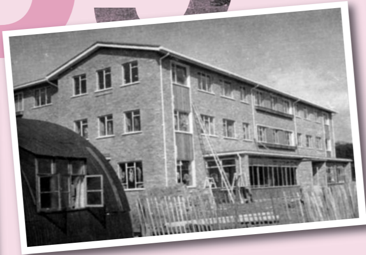
Hut at left is 17 (shortened to make room for the new building). Construction is almost complete.
