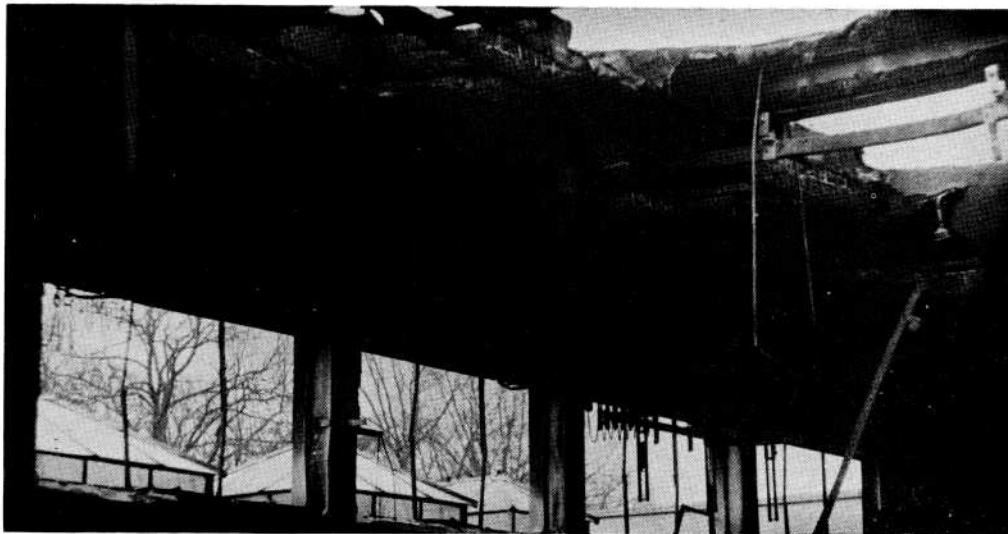
The Gym after the fire.
